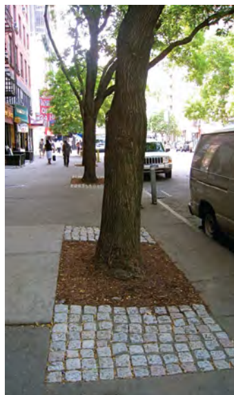
July 2010: 56 tree pits renovated as part of ongoing district street improvements.
